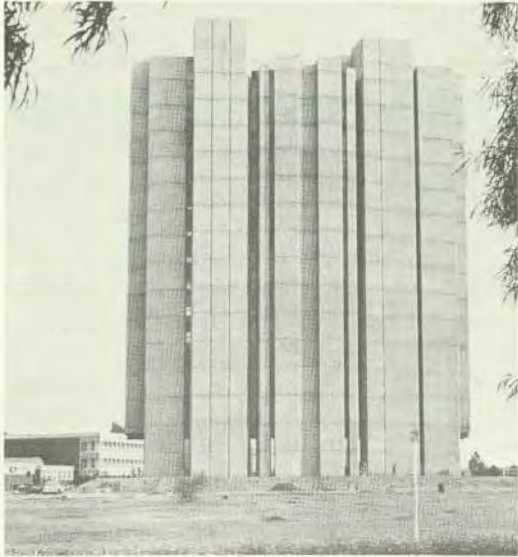
Diamant Sorting Building, Kimberley. Nordansicht
